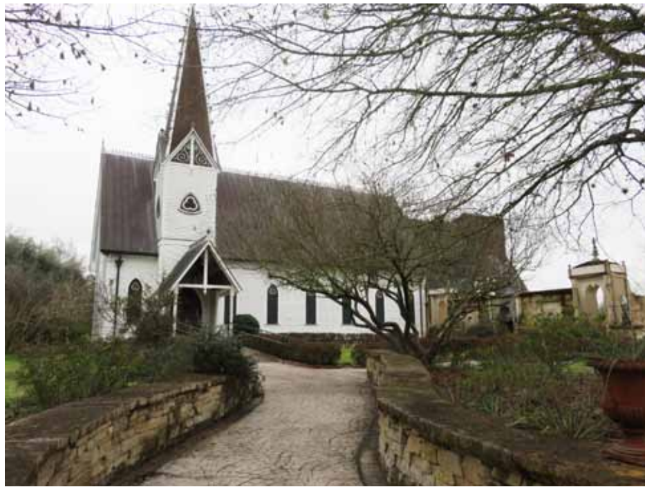
The Edythe Bates Old Chapel, built in 1883 and formerly the Travis Street United Methodist Church in La Grange, 16 miles away, was moved to the Round Top campus in 1994.
